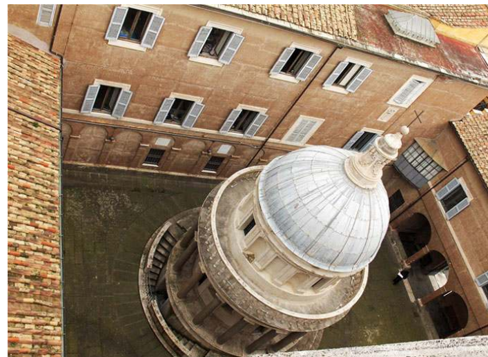
Royal Academy of Spain in Rome (Italy) – in progress
